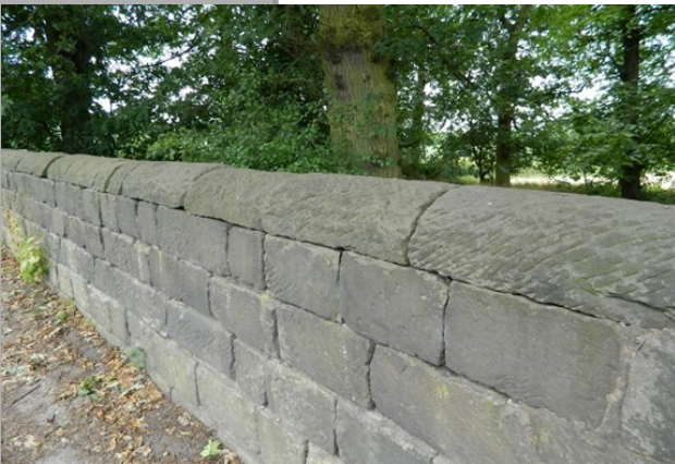
An old wall in Woodhouse
