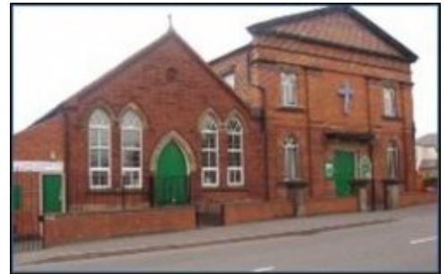
Methodist Church, Main Street
